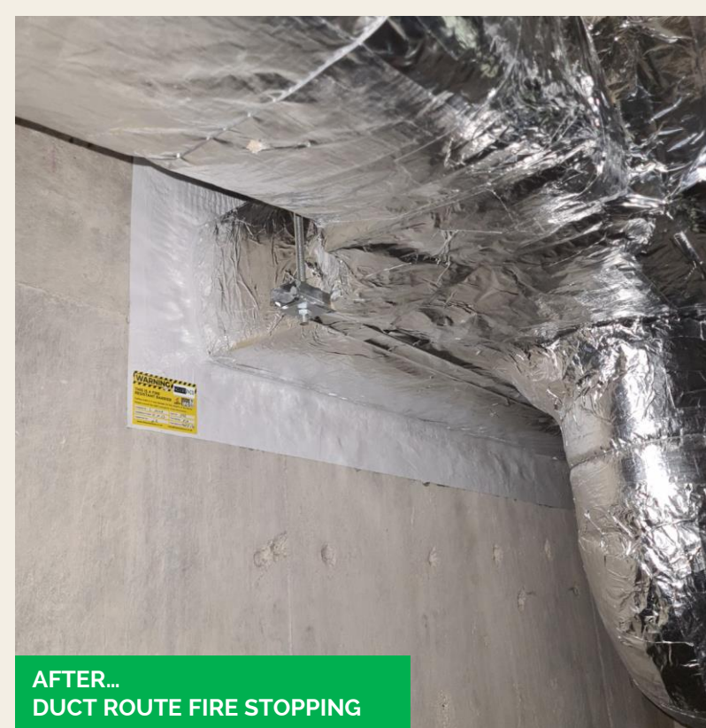
AFTER... PENETRATION FIRE STOPPING
