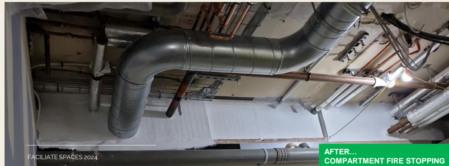
AFTER... DUCT ROUTE FIRE STOPPING
