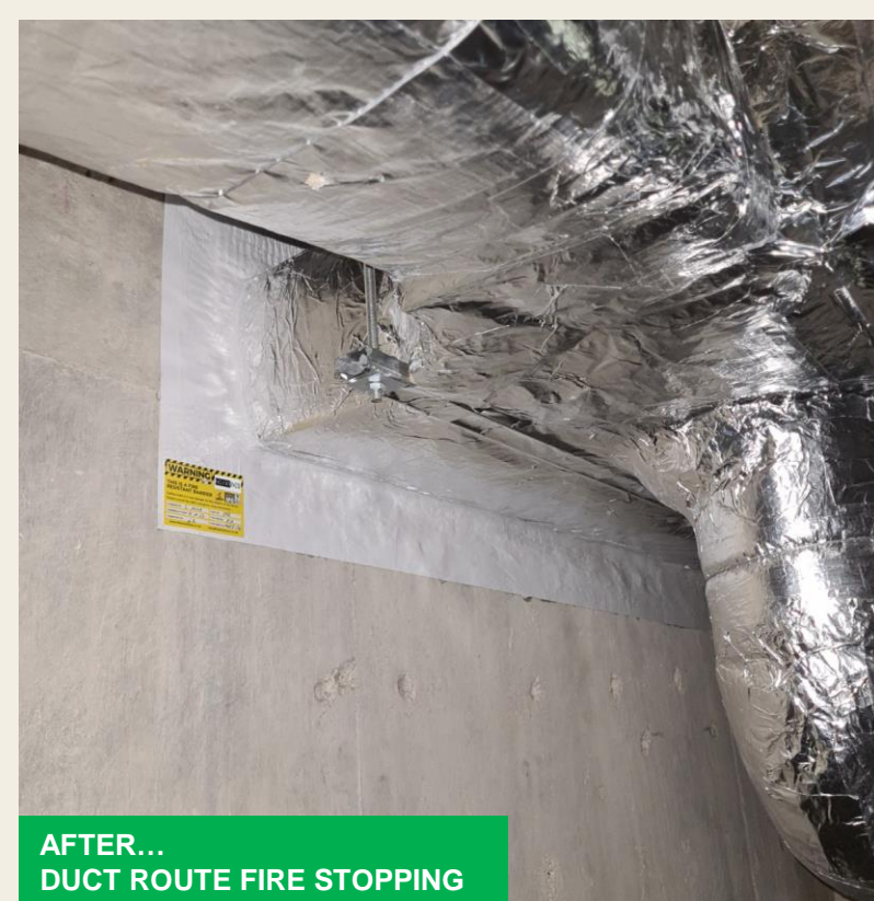
AFTER... PENETRATION FIRE STOPPING
